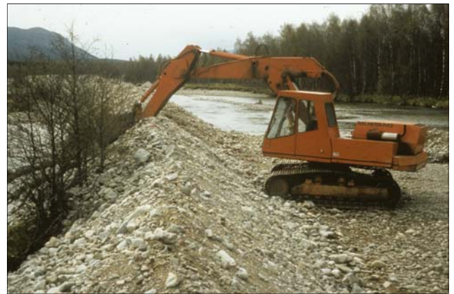
Digging the diverting channel.
